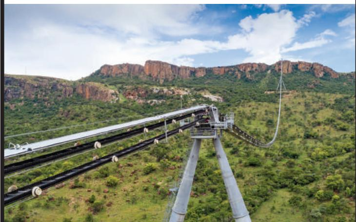
Australia’s DRA Global Ltd. (**No. 63**) is engineer to quadruple the capacity of the Booyensdal platinum mine for Northam Platinum in South Africa, including this three-mile rope conveyor using RopeCon technology.
