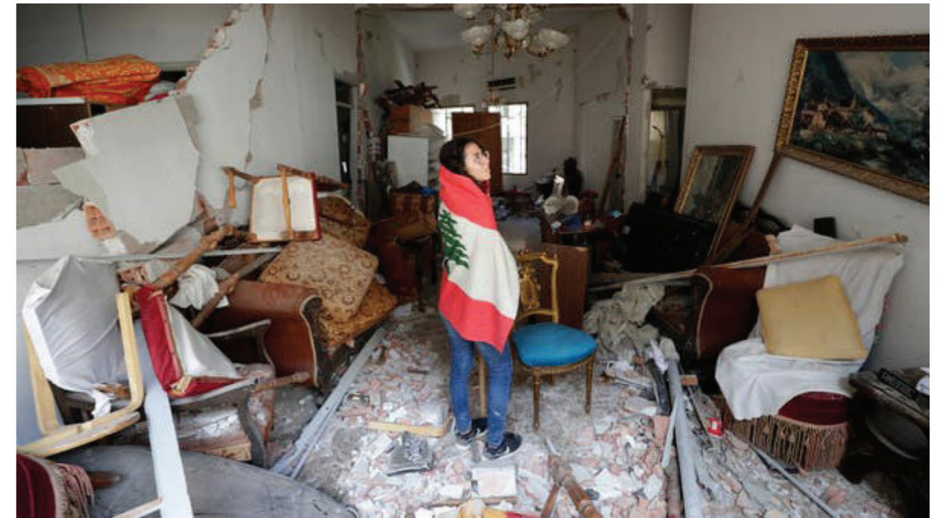
Figure 1.7. Damaged Apartments (Source: Emily Judd - Al Arabiya)
