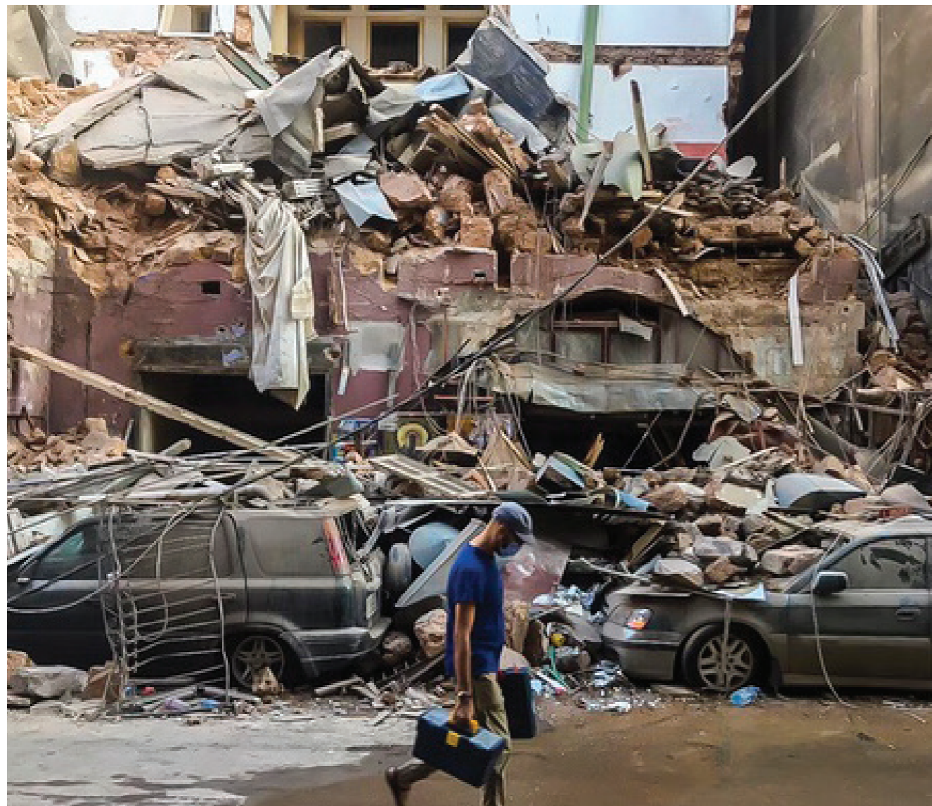
Figure 1.2. Damaged Building After Beirut Port Blast (Source Dalia Khamisy -British Red Cross)
